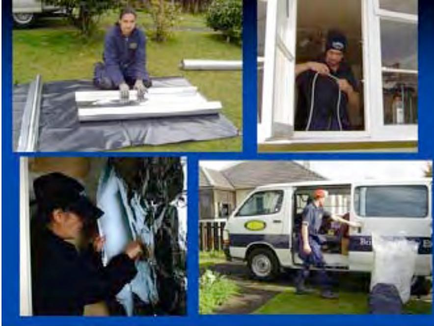
Community organisations such as the HEET Energy Efficiency Trust are involved in the retrofitting of older houses for energy efficiency, including installing underfloor and ceiling insulation to reduce heat loss.
