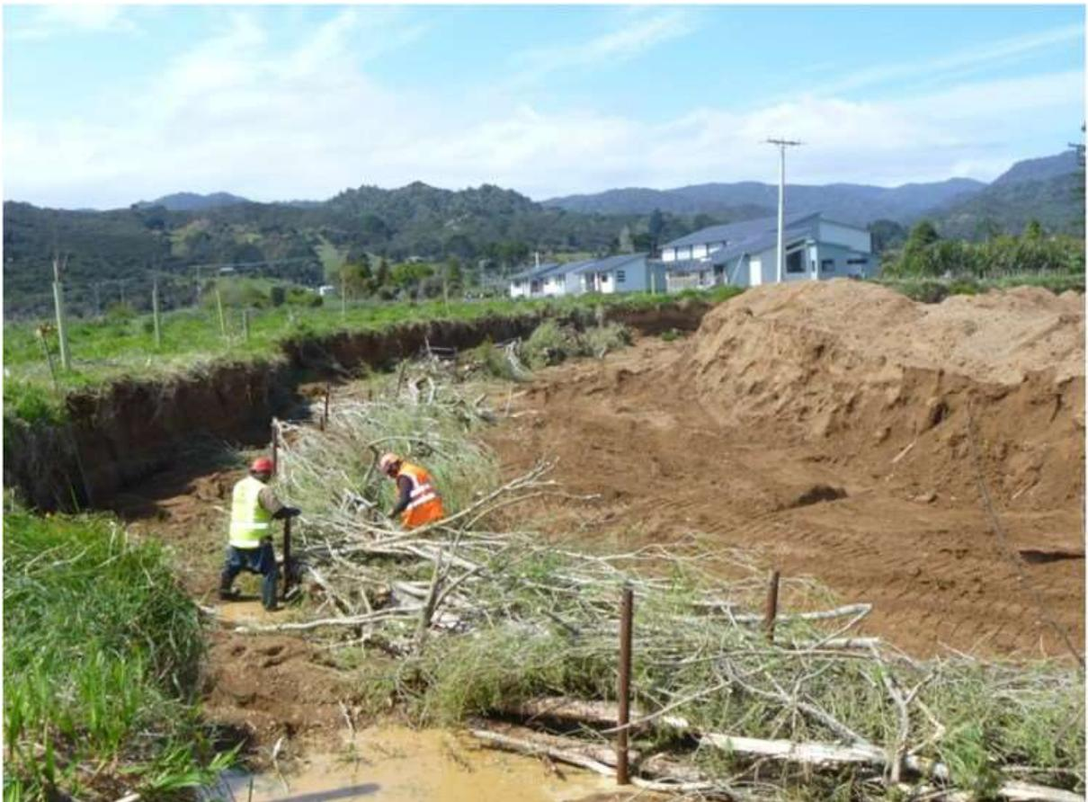
Picture 16 Stream bank erosion protection - tree tying or layering works as both erosion protection fish habitat
