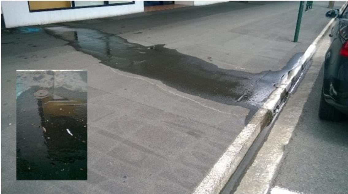
*Figure 30: Leaking urban water connection discharging potable water to the stormwater system*
